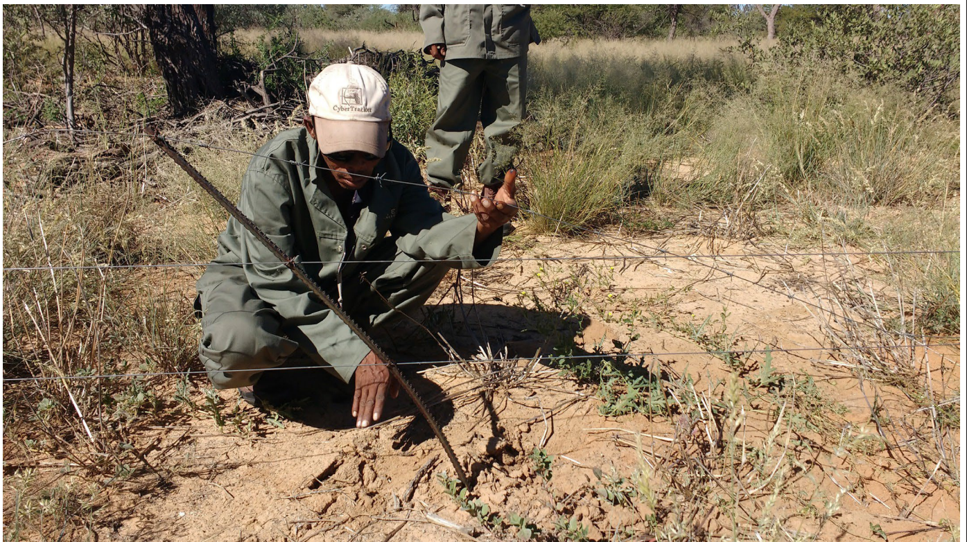
Figure 3) Master Tracker HL indicating where a gemsbok contacted the 'wildlife-friendly' fence, bending the metal fence post and damaging the top wire
